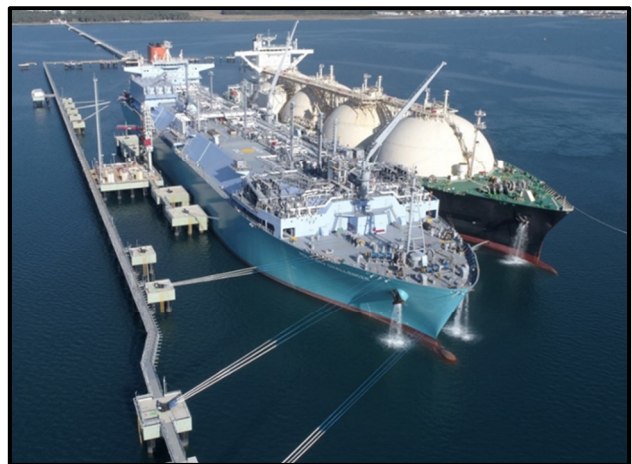
Figure 1, Typical high risk application, mooring
