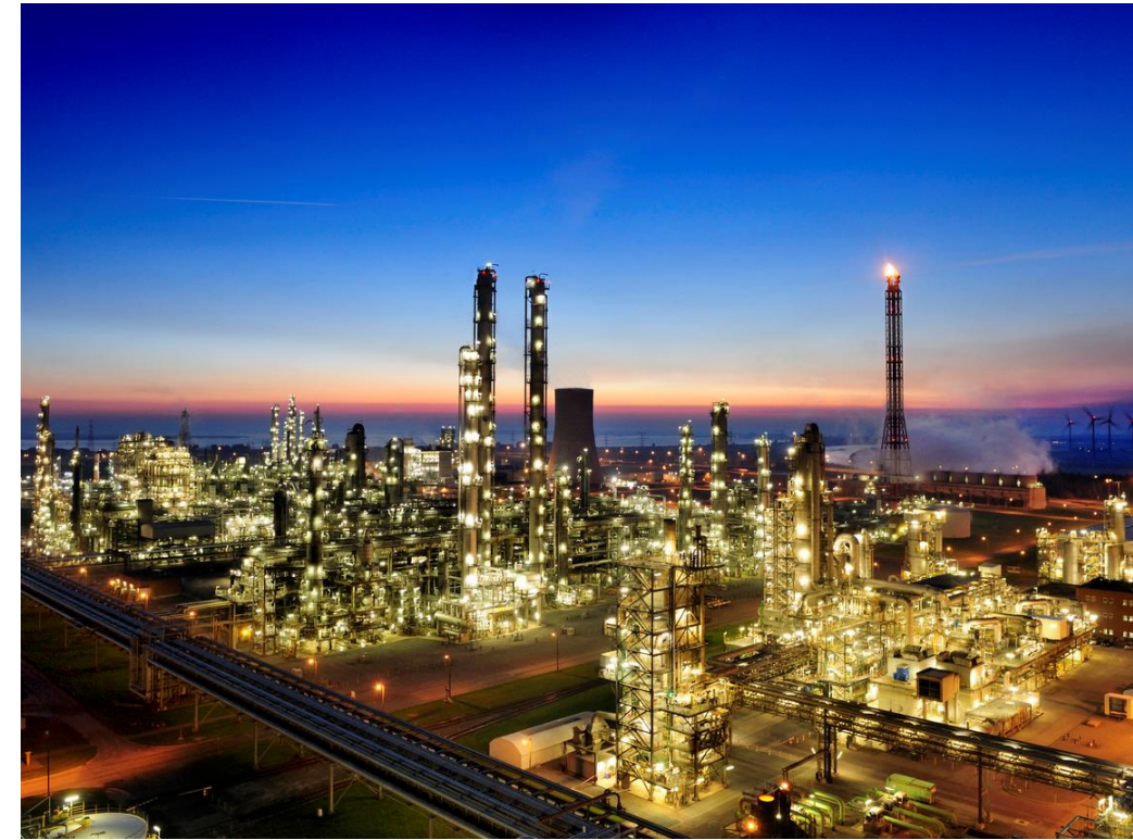
Illustrative picture of continuous production plant in BASF Antwerp
